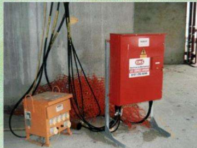
Rising Main Unit and Transformer
