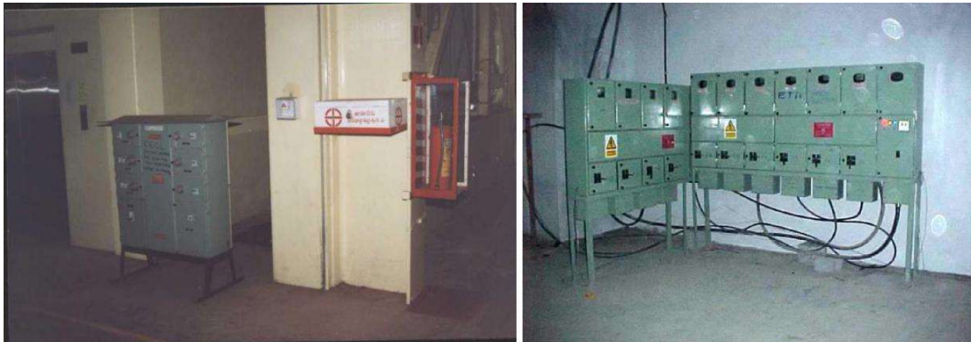
Rising Main Unit and Transformer
