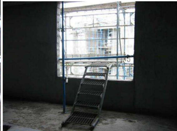
Proper Access to workplatform
